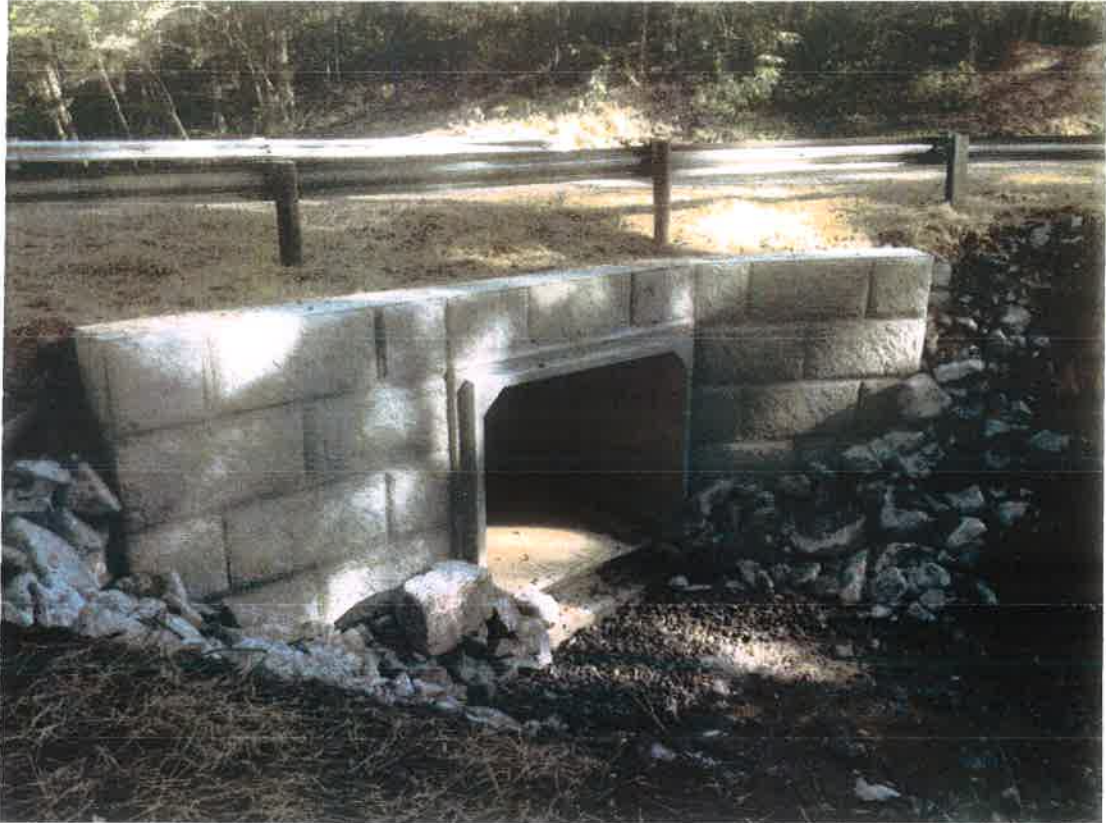
CR #32, Logan Horns Mill Road, 8' x 6' x 40' box culvert
